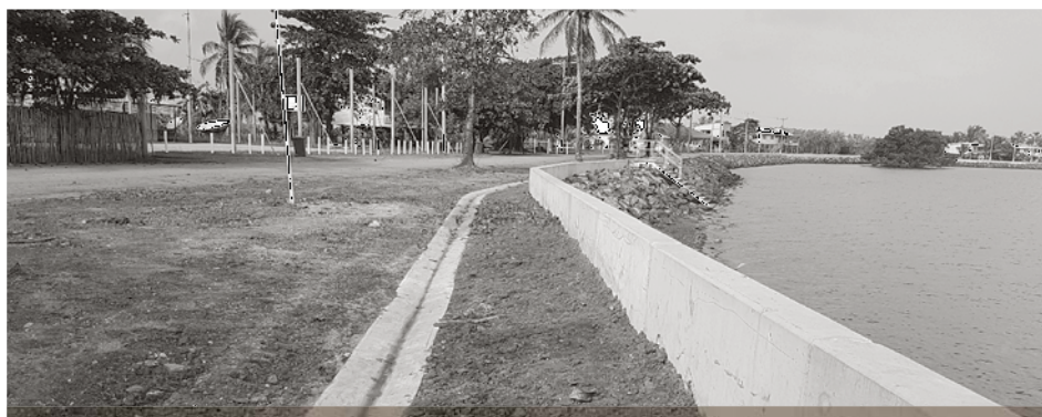
THE NEW SAIBAI SEAWALL.
