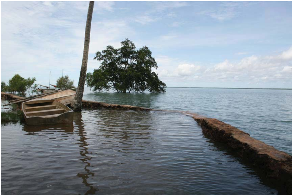
Photo 7. Saibai – community built seawall – January 2011 spring tide. (Source TSRA)
