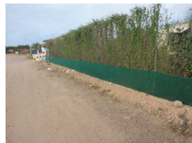
Installation of toad exclusion fence on Horn Island
