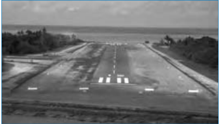
The bitumen sealed Warraber Airstrip.
