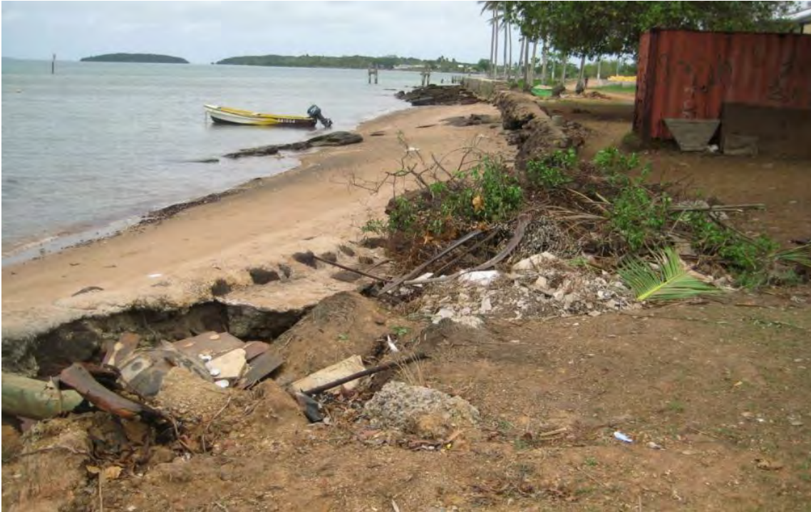
Figure 6 Rubbish used to fill piping failure holes.
