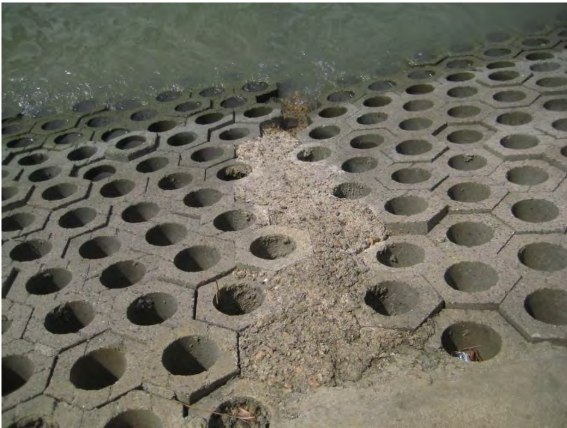
Figure 22 Junction in Seabee seawall
