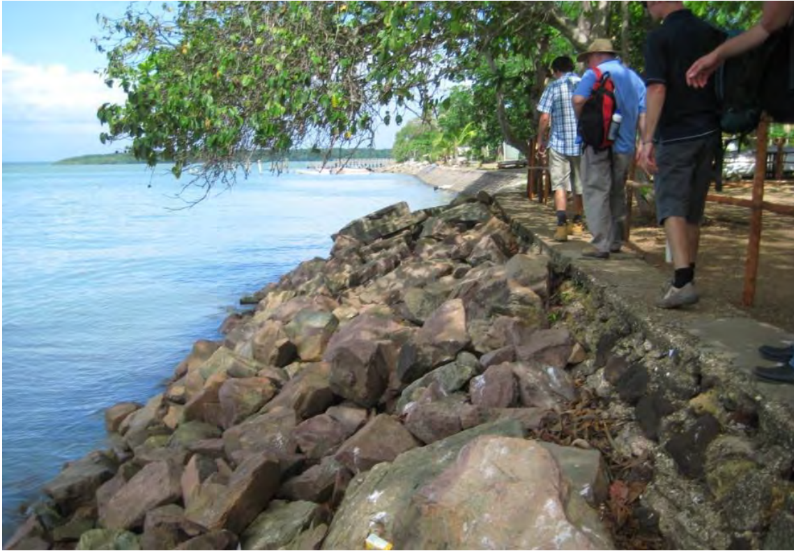
Figure 20 Rock armour seawall built over a relic block work wall
