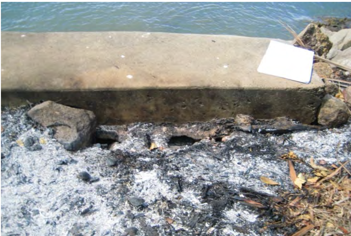
Figure 24 Crest of wall with gap behind the capping beam
