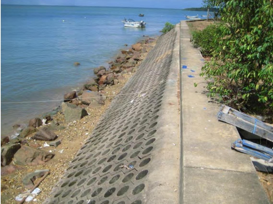
Figure 29 Armoured toe for Seabee seawall.
