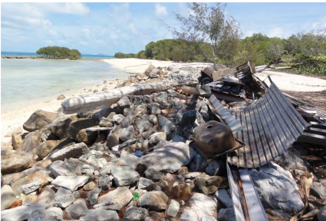
Figure 45 Northern end of seawall (note rubbish piled up to reinforce seawall crest)
