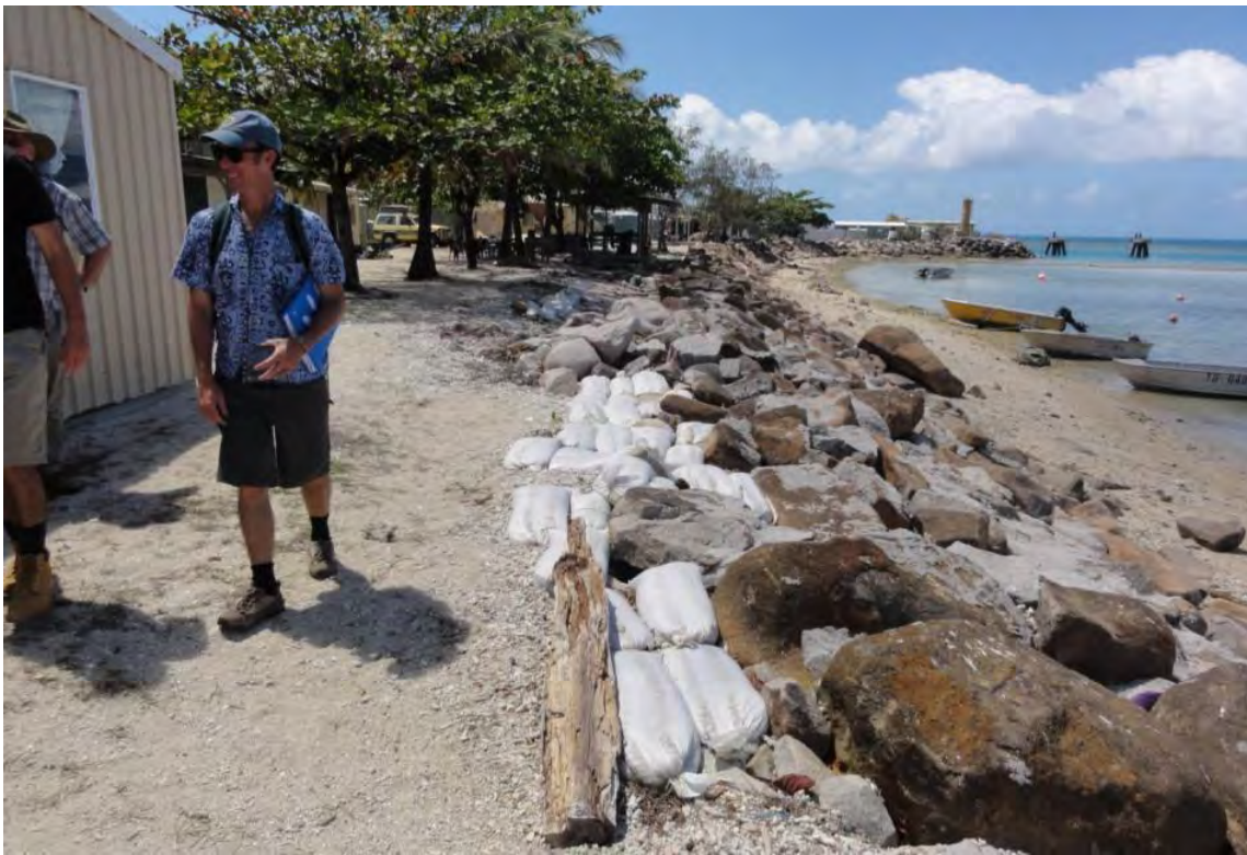
Figure 46 Sand bagging to stabilise areas behind seawall
