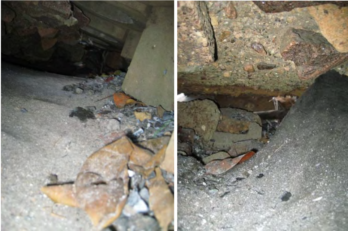
Figure 25 Beneath armour; note Seabee settled onto sand (l) & Figure 26 capping beam undermined (r)
