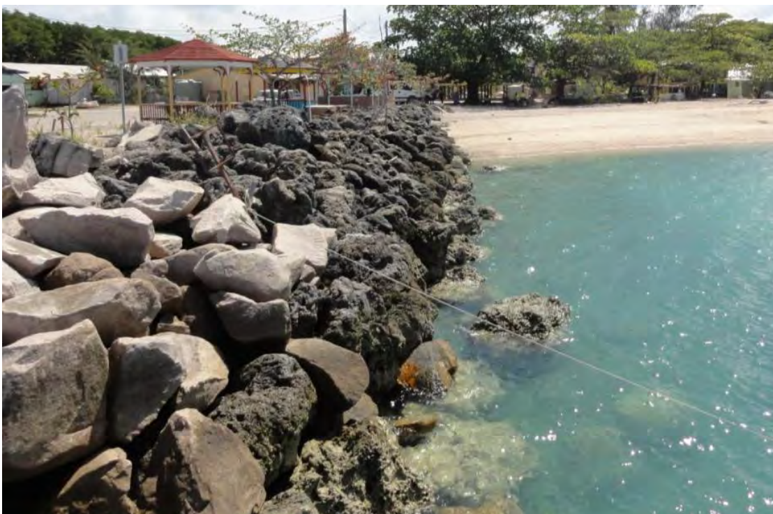
Figure 54 Rock armour seawall on Iama Island (note the native rock in foreground and the coral rock beyond)
