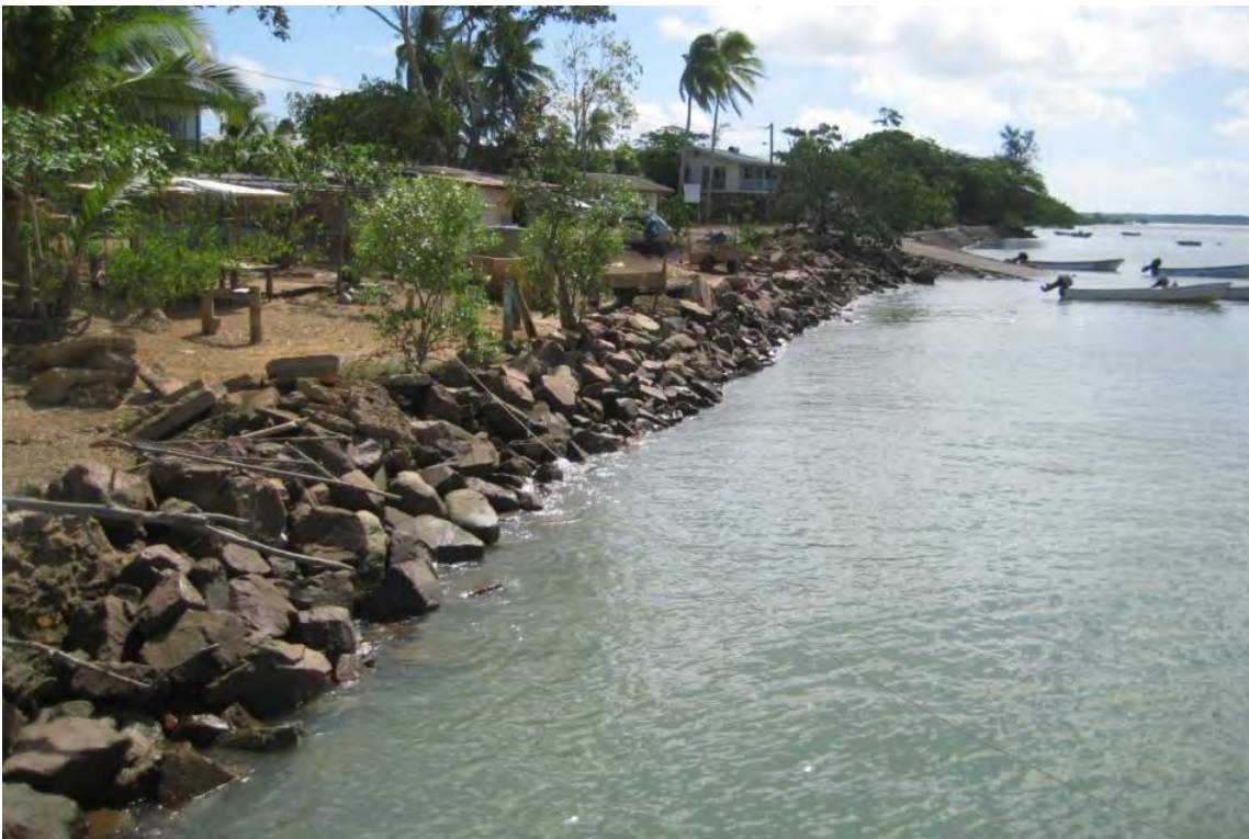
Figure 28 Inadequate seawall looking west towards boat ramp (note mangrove trees behind seawall)
