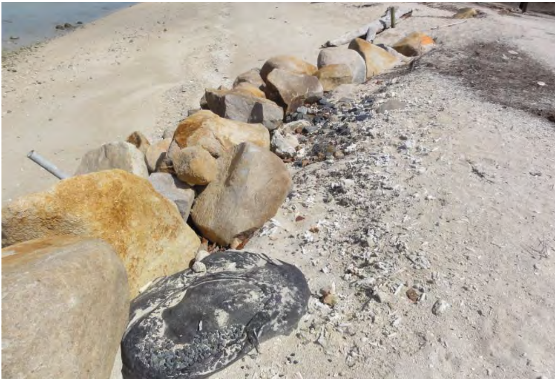
Figure 35 Slumped section of the seawall
