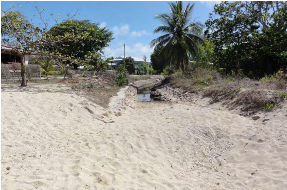
Figure 38 Lined channel discharges onto beach
