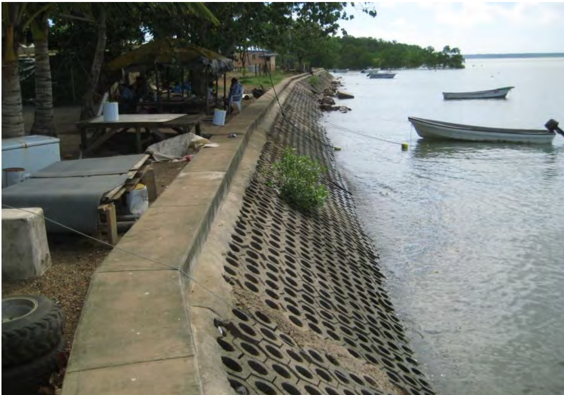
Figure 21 Seabee seawall in good order (note mangrove growing out of wall)
