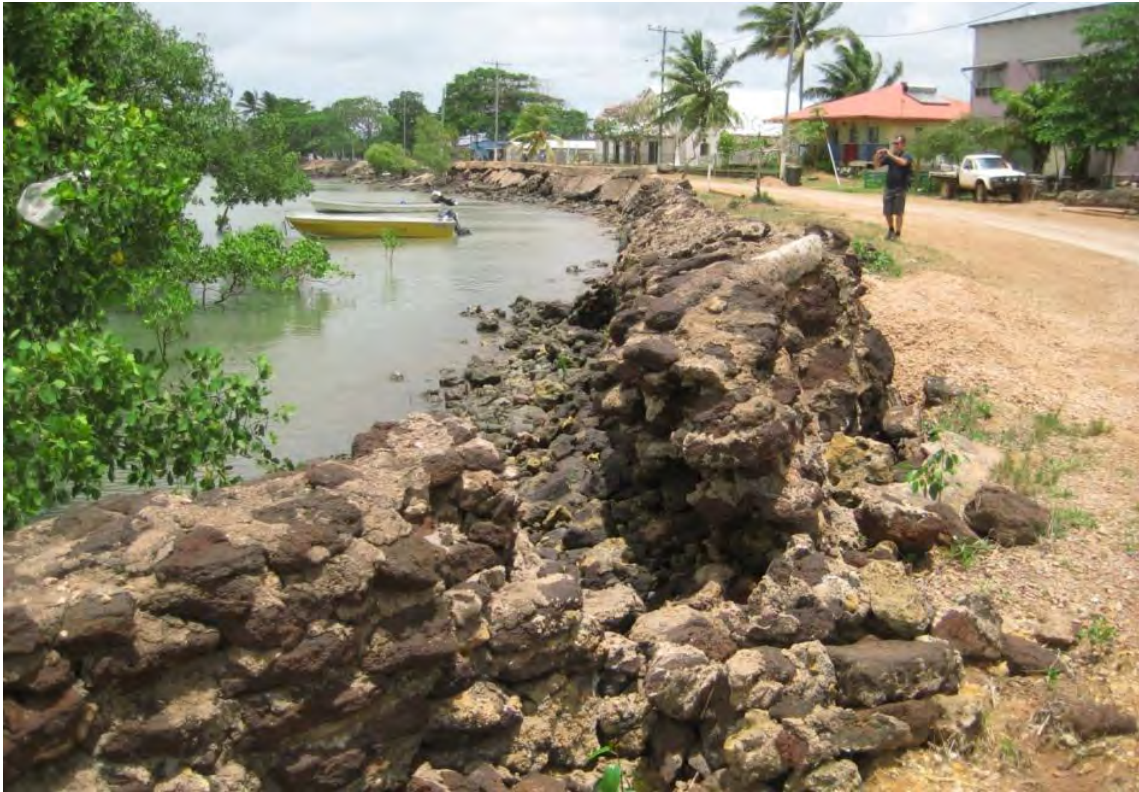
Figure 9 Localised failure (foreground) probably due to overtopping and piping more distant front face failure due to undermining of toe
