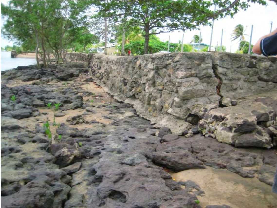
Figure 10 Section of wall with large cracks, ready to collapse seaward during high wave/water level event.
