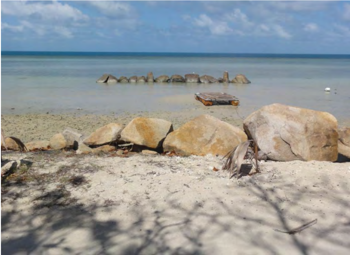
Figure 36 Ineffective offshore breakwater
