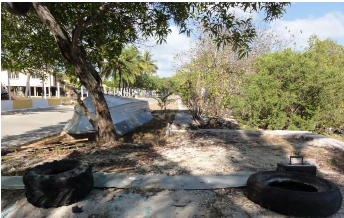
Figure 50 Double line of defence, low wall facing mangroves and higher yellow/white wall protecting houses (I).
