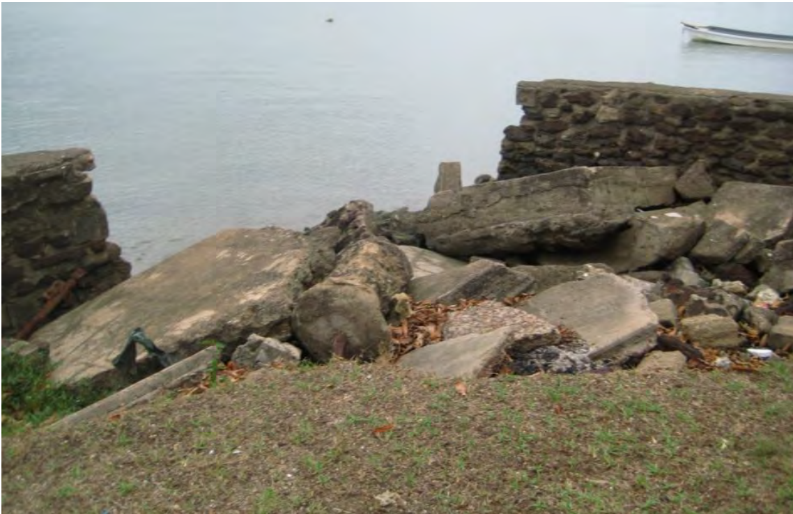
Figure 7 Failure (collapsed landward) due to piping and toe undermining
