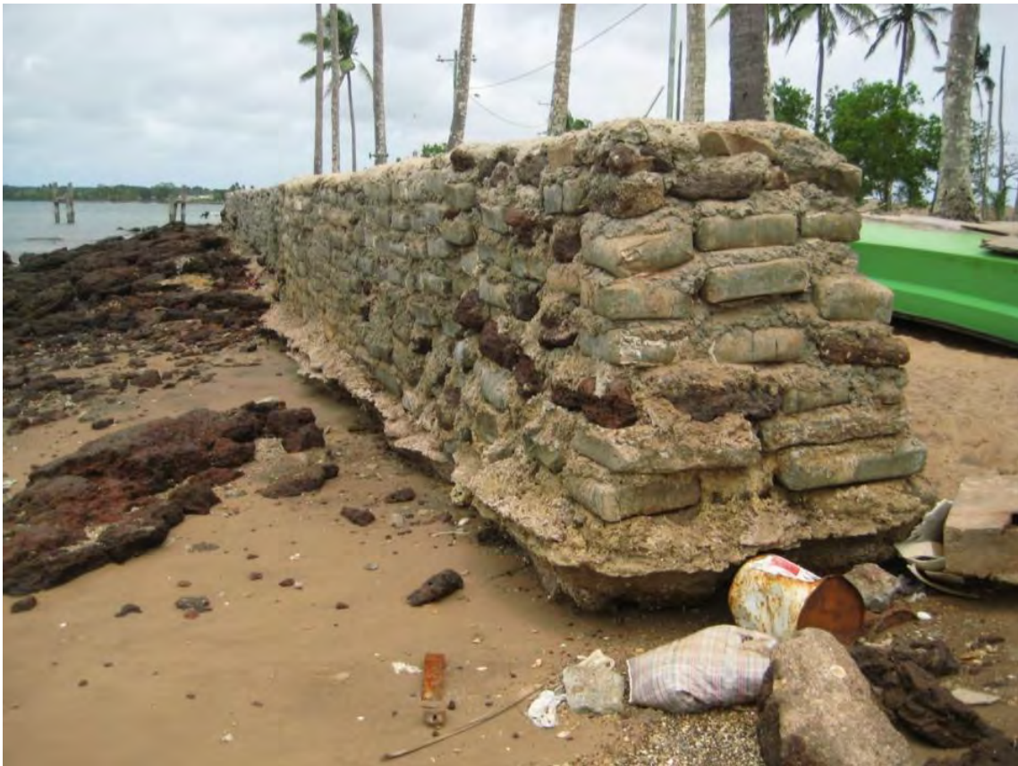
Figure 3 Example of toe undermining
