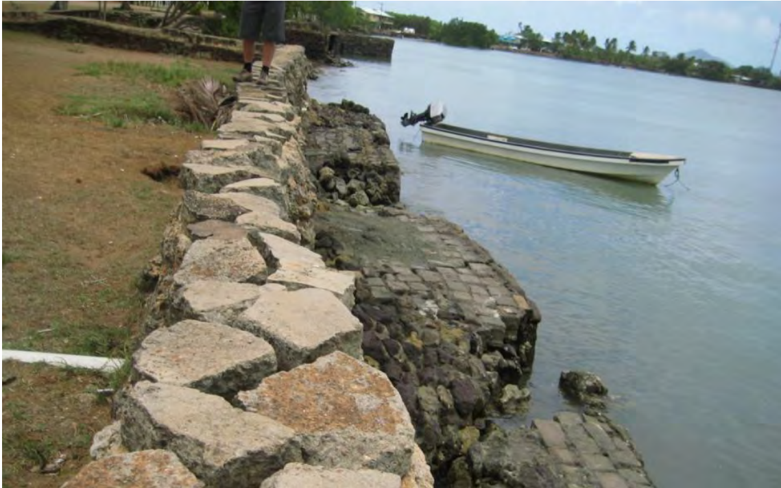
Figure 8 Failure (old wall collapsed seaward) due to toe undermining
