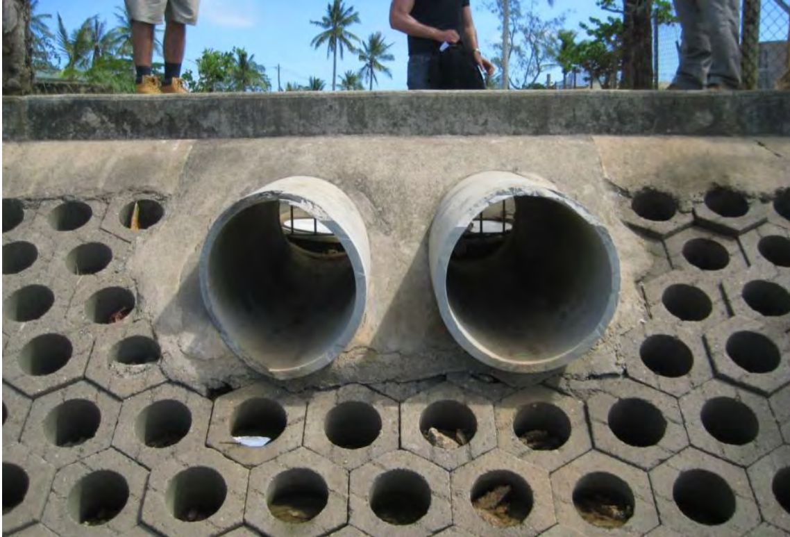
Figure 30 Drains through seawall have lost gates and allow back flooding.
