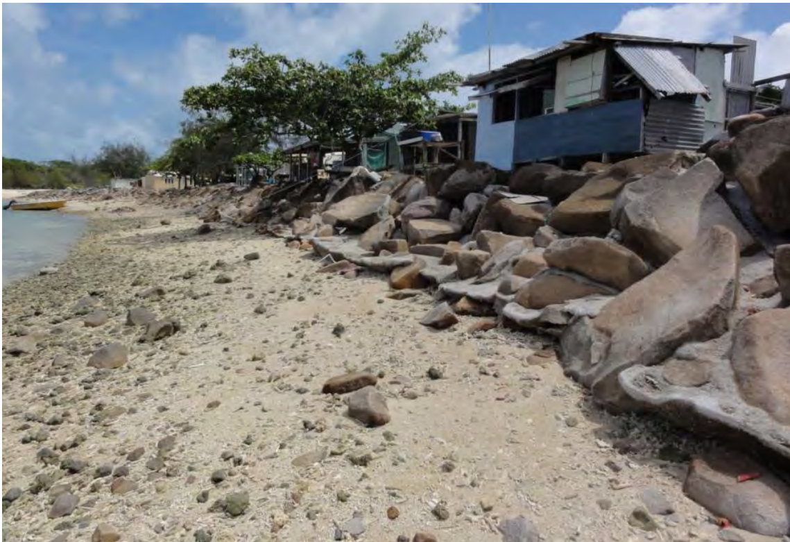
Figure 44 Northern beach seawall undermined by beach erosion.
