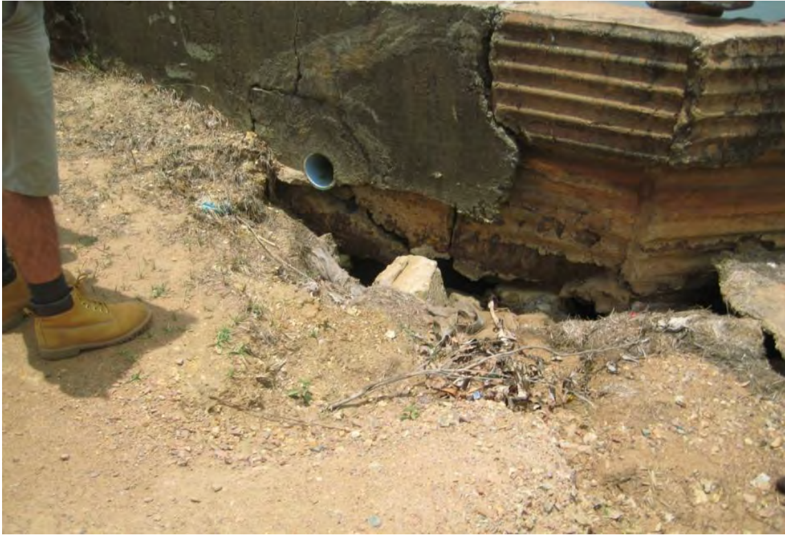
Figure 4 Example piping failure
