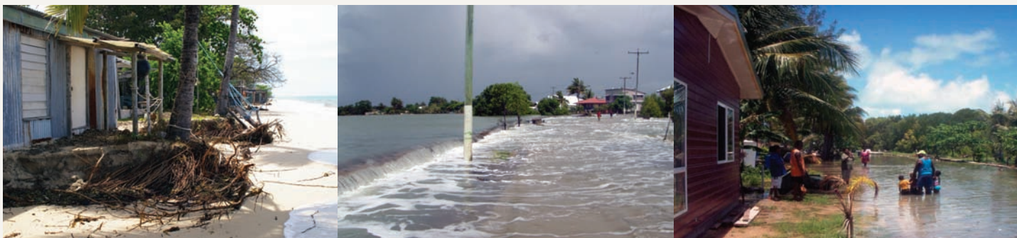
Erosion on Masig Jan 2009 Photo: Annick Thomassin
