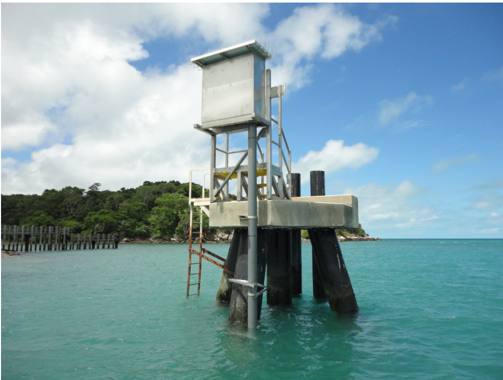
Caption: Tide gauge housing now installed at Kubin, Moa Island for monitoring of rising sea levels (Image: TSRA).
