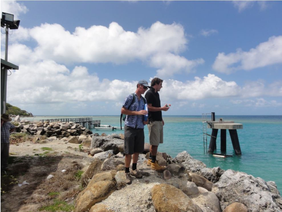
Caption: TSRA Coasts and Climate Project Manager John Rainbird with an engineer assessing the seawall at lama (Yam Island) (Image: TSRA).
