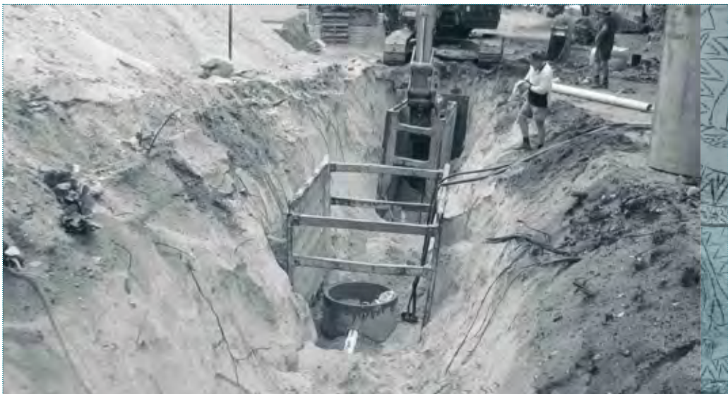
Above: Warraber Sewer - Trench digging.
