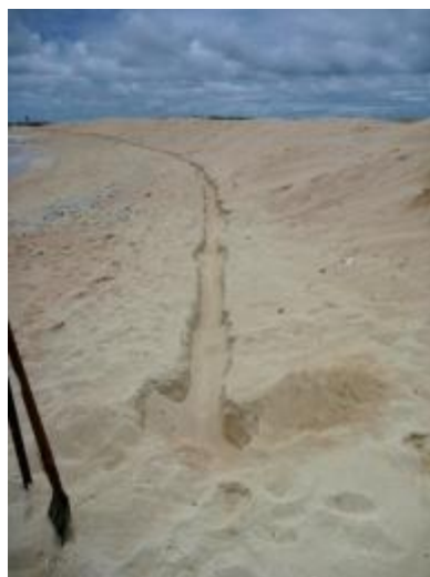
Figure 24: The 75m excavated trench on the northern shoreline of Maizab Kaur February, 2015.
