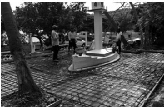
RANGERS AND WORKERS FROM MY PATHWAY AND STRAIT SUPPORT PREPARING THE COMING OF THE LIGHT MONUMENT SITE FOR CONCRETING
