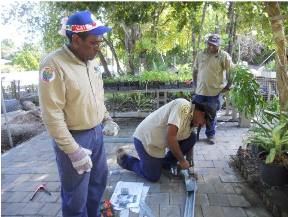
Caption: Ugaram Ranger Noel Baker and Erubam Ranger Aaron Ketchell erecting the frame of the new shed for Mothers Well Nursery with Regional Landcare Facilitator George Saveka looking on. (Image: TSRA)
